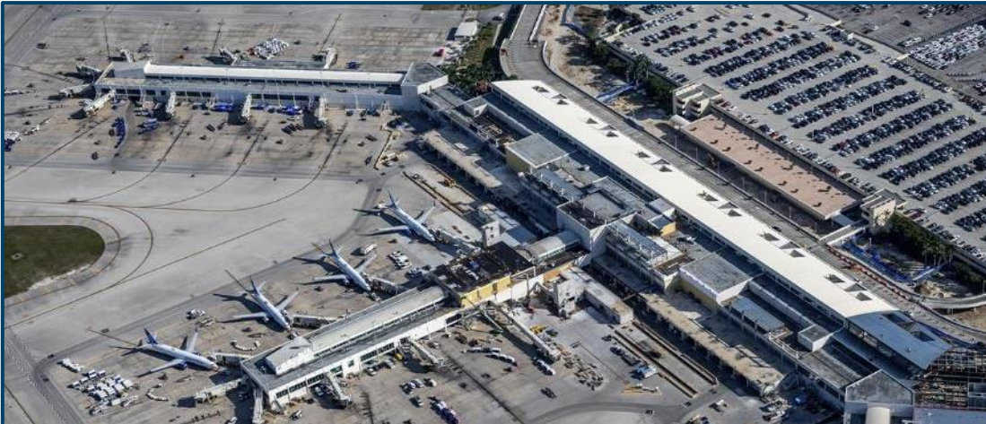
RSW Phase I: Aerial Looking SE
