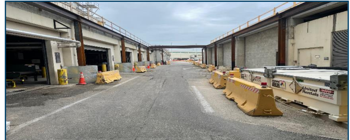
Looking west from Concourse C: Steel Beam Prep for Hollow Core
