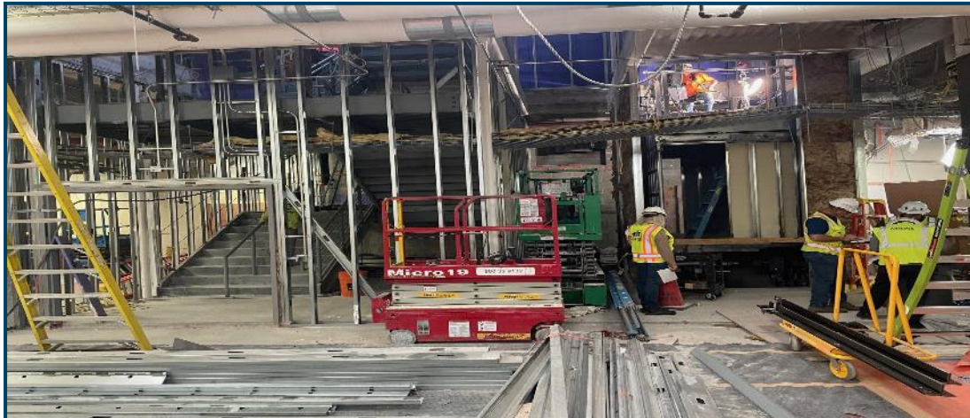
Zones 5 & 6: New Stairwell (installed) & Elevator Core (ongoing)
