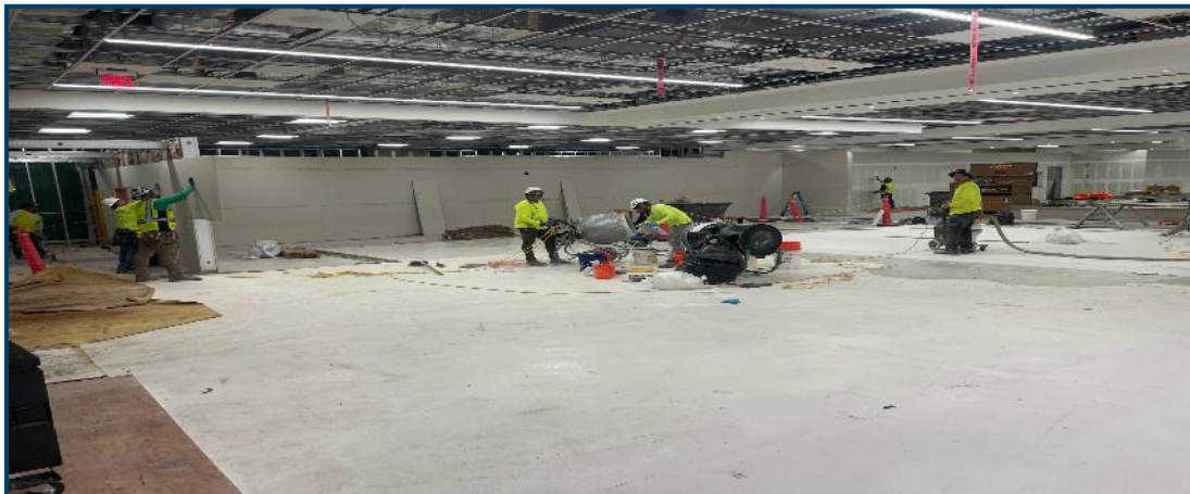
Concourse C: Temporary Checkpoint – Framing to Passenger Bridge
