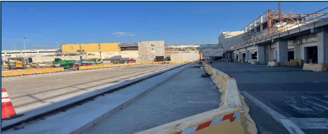
Looking east to Concourse C: Tower Crane Foundation Complete
